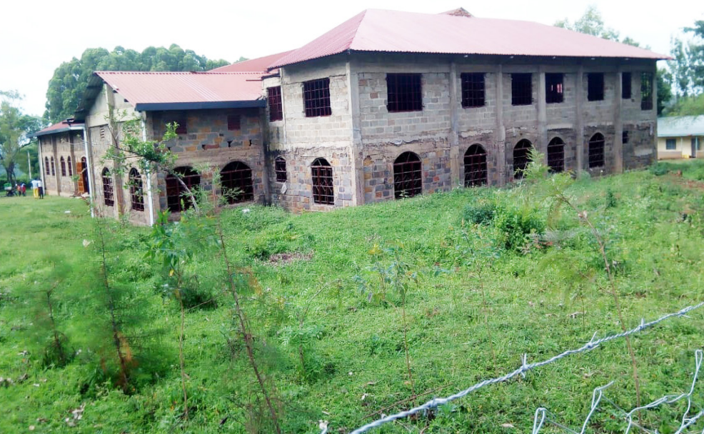
St. Pauls Memorial Church Maseno under Construction
