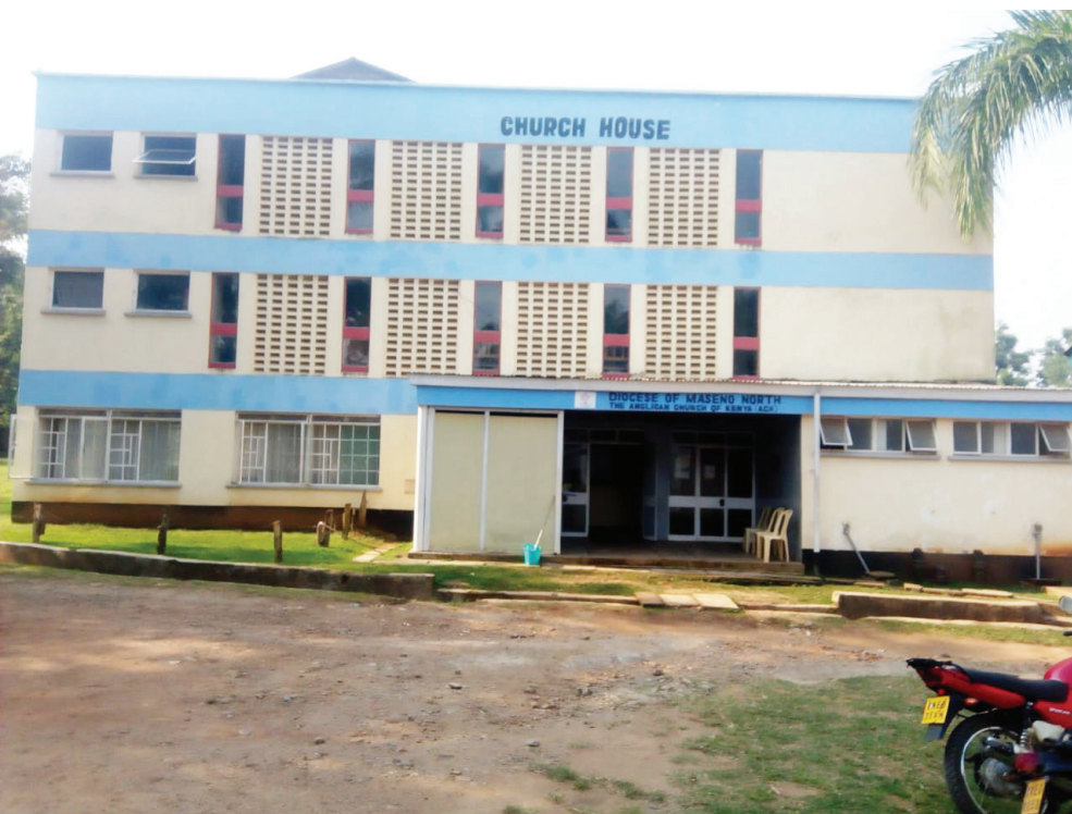
ACK Diocese of Maseno North Administrative Office, Kakamega
